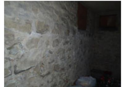
*CONDITION:* Staining was observed: Evidence of prior water penetration is noted- Seen under windows and at some corners.
