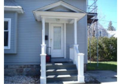
*TYPE:* Treated deck top and substructure.
