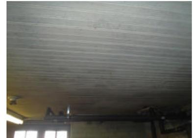
*FLOOR JOIST TYPE:* 2x10.
