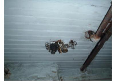
Several live knob and tube circuits noted - recommend contracting an electrician to get an estimate to update the wiring.
