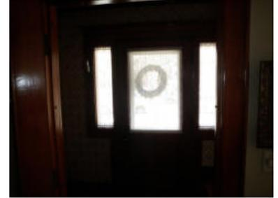
Left side door; action needed, glass is cracked and has a major bow. Recommend having this repaired before the leaded glass falls out.
