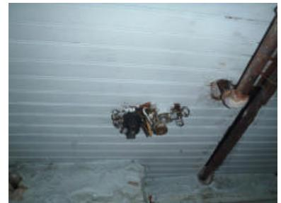
Several live knob and tube circuits noted - recommend contracting an electrician to get an estimate to update the wiring.
