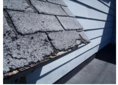
Margins between tabs are spreading indicating the shingles are at the end of their life.
