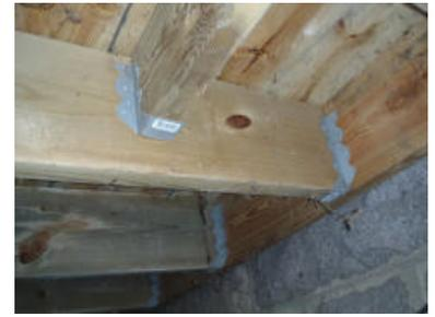
*FLASHING* Due to very limited viewing, we cannot determine whether or not flashing has been installed between the ledger and the rim joist. This area is very prone to moisture damage and hidden damage should not be a surprise if this area is not flashed or improperly flashed.
