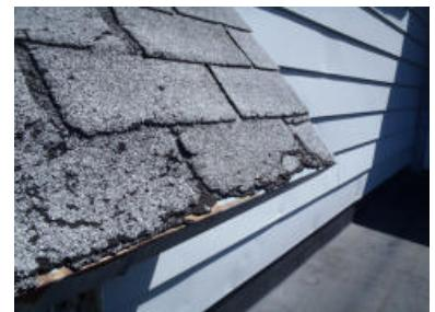
Margins between tabs are spreading indicating the shingles are at the end of their life.
